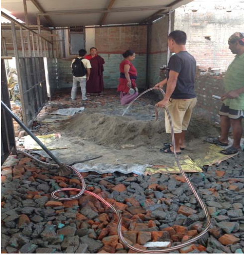
Foundations being laid for three new semi permanent classrooms
