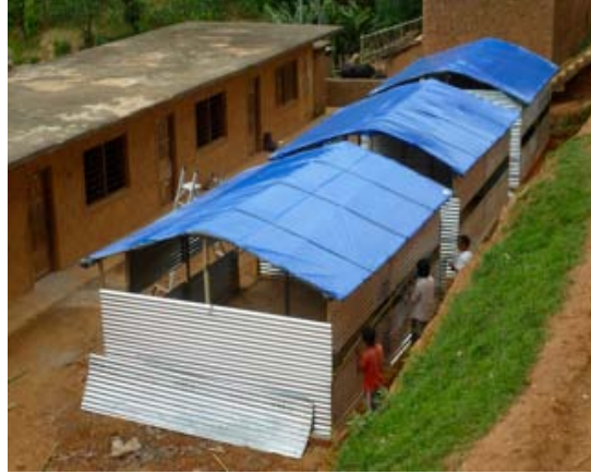
Construction of 3 classrooms
