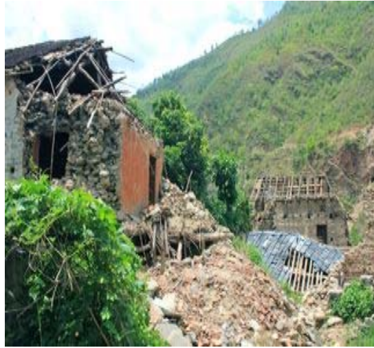
So much damage
