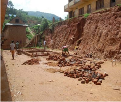
Foundations being laid
