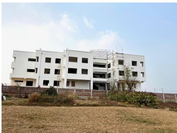
Construction of the Siddhasthali Rural Community Hospital
