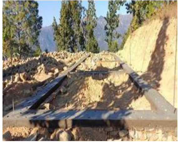
Foundations being dug
